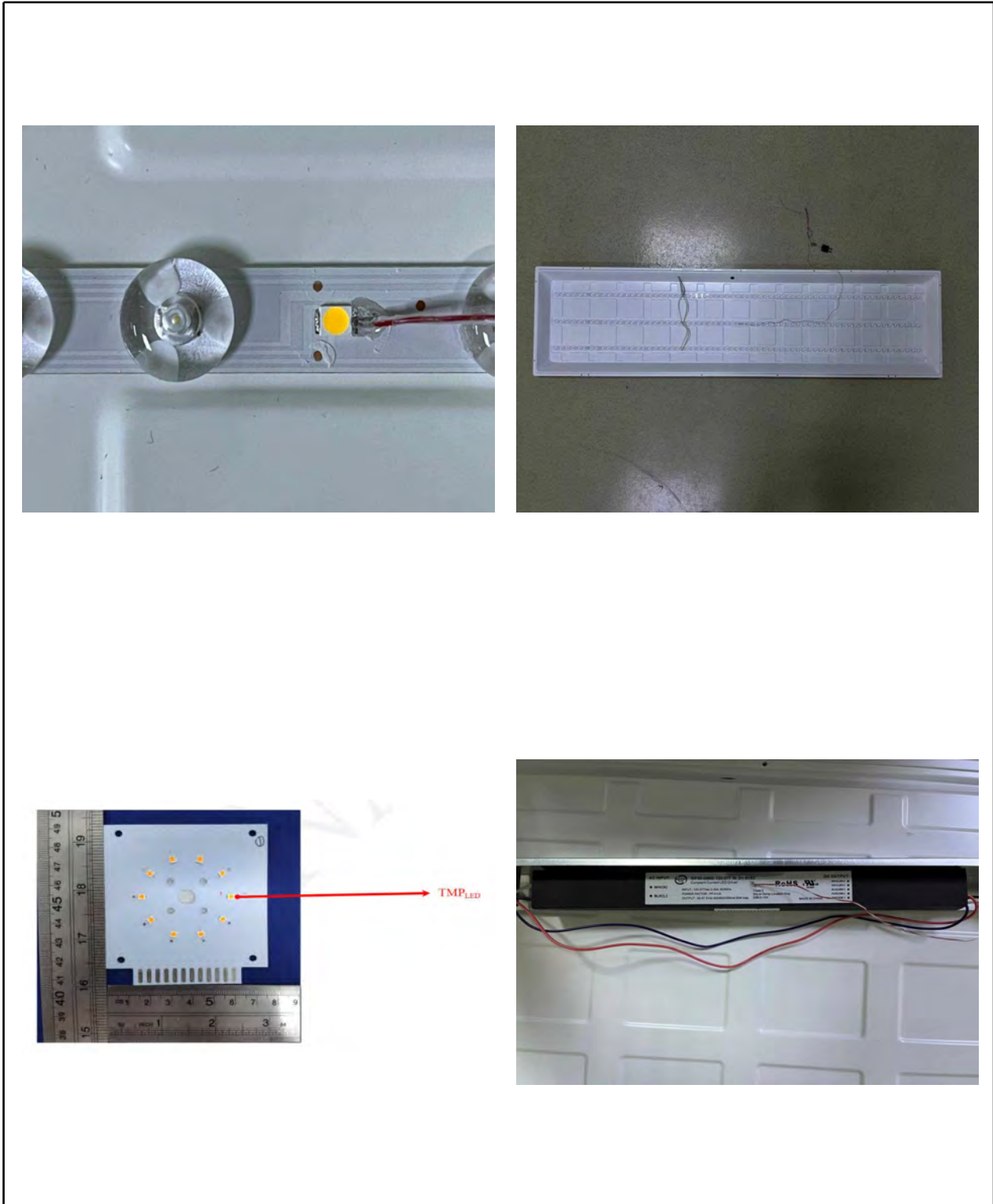
Test Photos for Ts Point of Light Sources & Tc Point of Drivers
