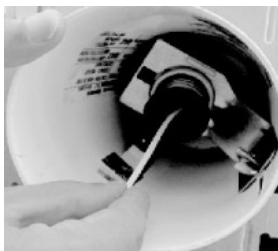
STEP 2: Twist adaptor into socket
