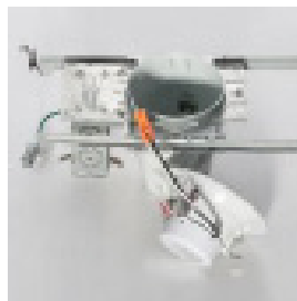
STEP 3: Insert male connector into female one.
