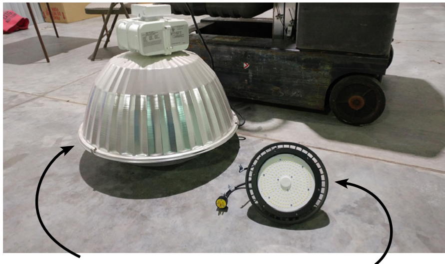
HID FIXTURE BEFORE &amp; COMPASS HIGH BAY AFTER
