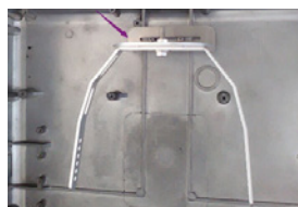
Shoe Box/Flood/Area Fixture Installation
