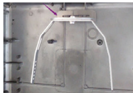
Shoe Box/Flood/Area Fixture Installation
